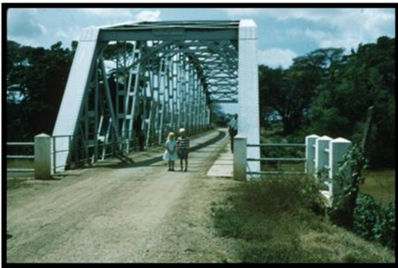
Figure 4a: Araara Bridge built by Antonio Badoni SpA in the 1930s. Now it is totally destroyed.
